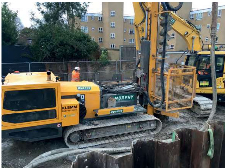
A KLEMM KR 709-3G, supplied by Skelair International to J. Murphy & Sons, in operation at Iver station, London
